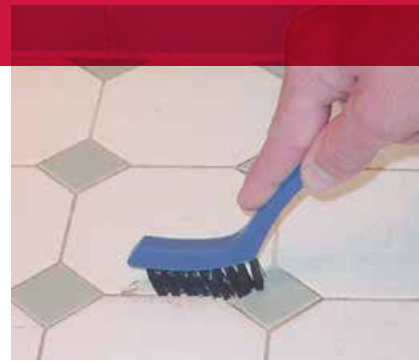
Removing stubborn dirt, grime and mildew from a tiled surface with a grout detail brush.
