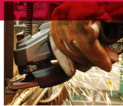
Blending fillet welds to ensure proper penetration prior to inspection.
