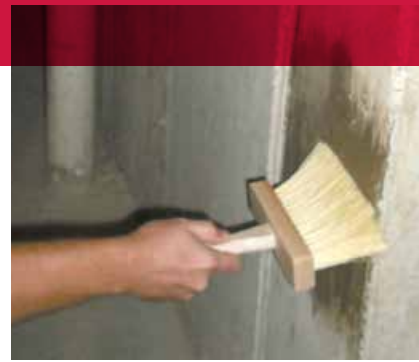
Applying waterproofing material with a masonry brush.
