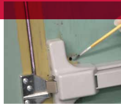
Painting a tight area on a steel door with a Marking Brush.
