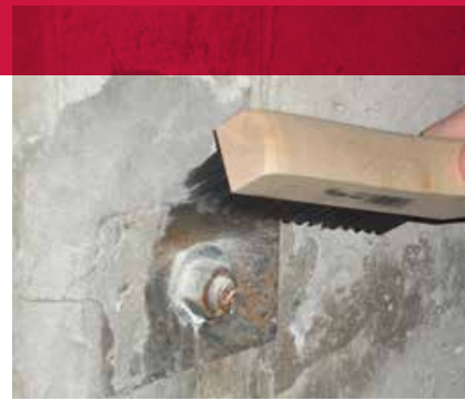
Removing excess concrete from the surface of a steel support plate.
