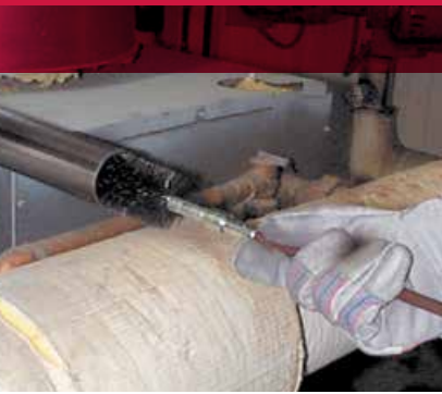
Cleaning boiler pipes with a flue brush.
