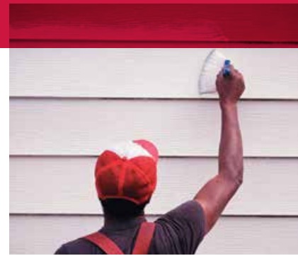
Applying paint to clap board siding.
