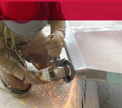
Grinding on a platform for weld preparation.
